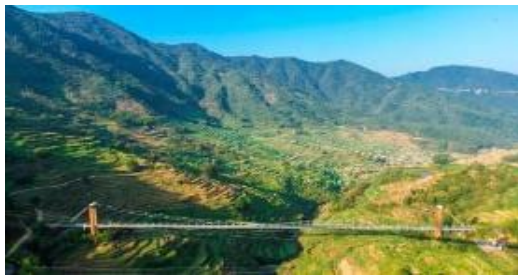
Wuyuan Glass Bridge
