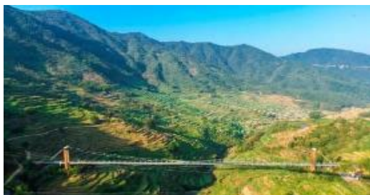
Wuyuan Glass Bridge
