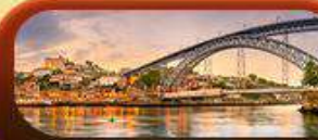
DOM LUIS I BRIDGE
