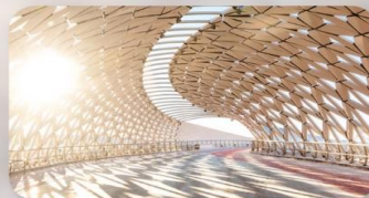
Atyrau Bridge Astana
